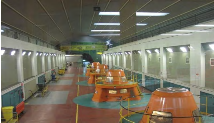
Tumut 1 Power Station
