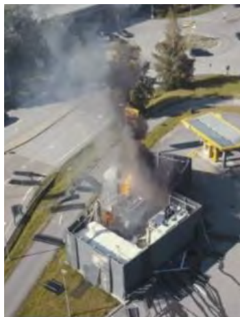
Hydrogen filling station aflame, Norway
